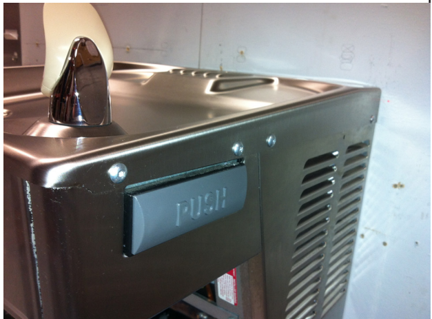
Fasten Basin Assembly in place.
