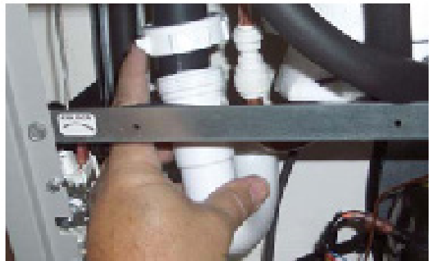
Reattach drain line to P-trap
