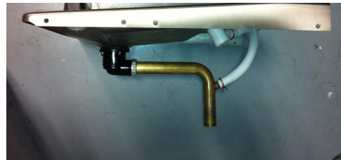
Exchange Drain hardware.
