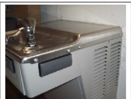
Remove Basin Fasteners
