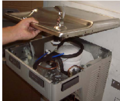
Lift and Remove Basin.
