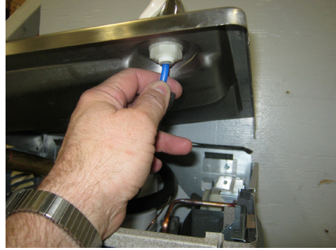
Remove Bubbler Water Line
