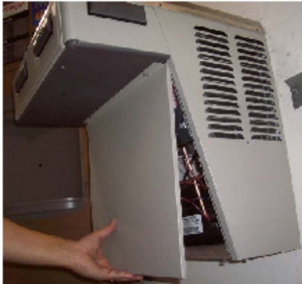
Remove Front Panel
