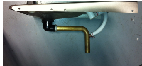
Exchange Drain hardware.
